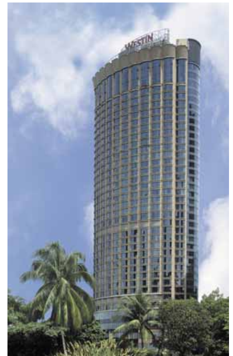
The Westin Kuala Lumpur has successfully combined five-star facilities with the latest technology from Clipsal Integrated Systems.
